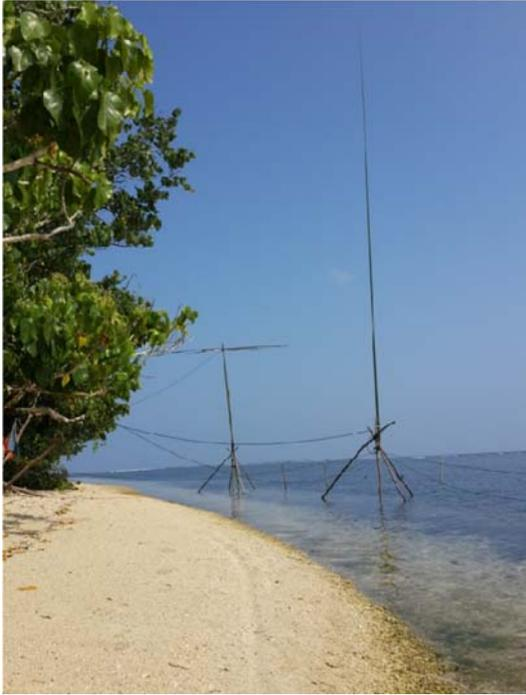
The next job is to attach the antenna to the mast of the bamboo plant and some branches of wood as a buffer so that the antenna can stand. This job is quite difficult because the ground is the sand and stones. Finally at 13.00 noon all antennas can stand perfectly.
