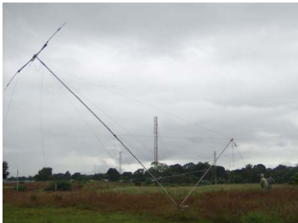
Erecting the 2el Tribander – the PA3AN way
